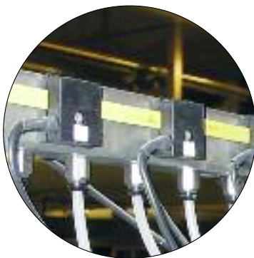
AS-Interface vampire contact for the control module ⇨ BUS
